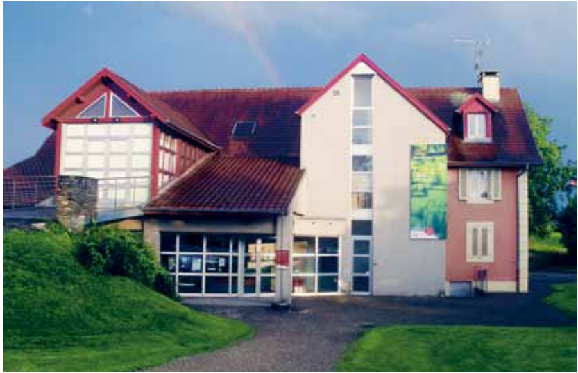
Espace multimédia gantner, view of front entrance with rainbow Photo © Espace multimédia gantner Photo: Fabien Velasquez
